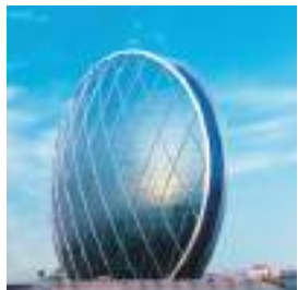
Aldar HQ Abu Dhabi
